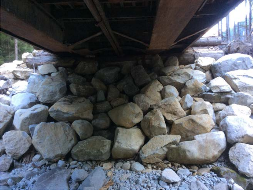
Right Bank Abutment when facing downstream
