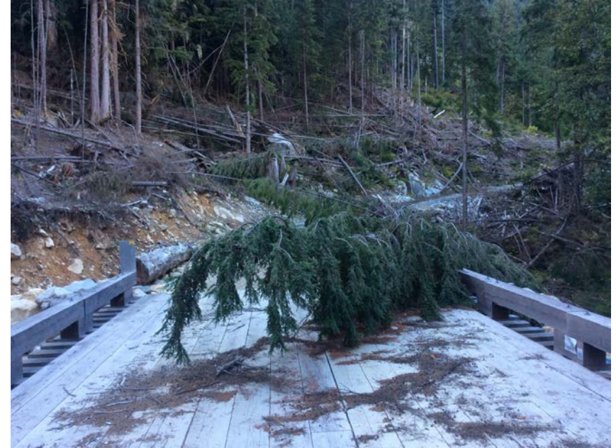
Left approach viewed from bridge
