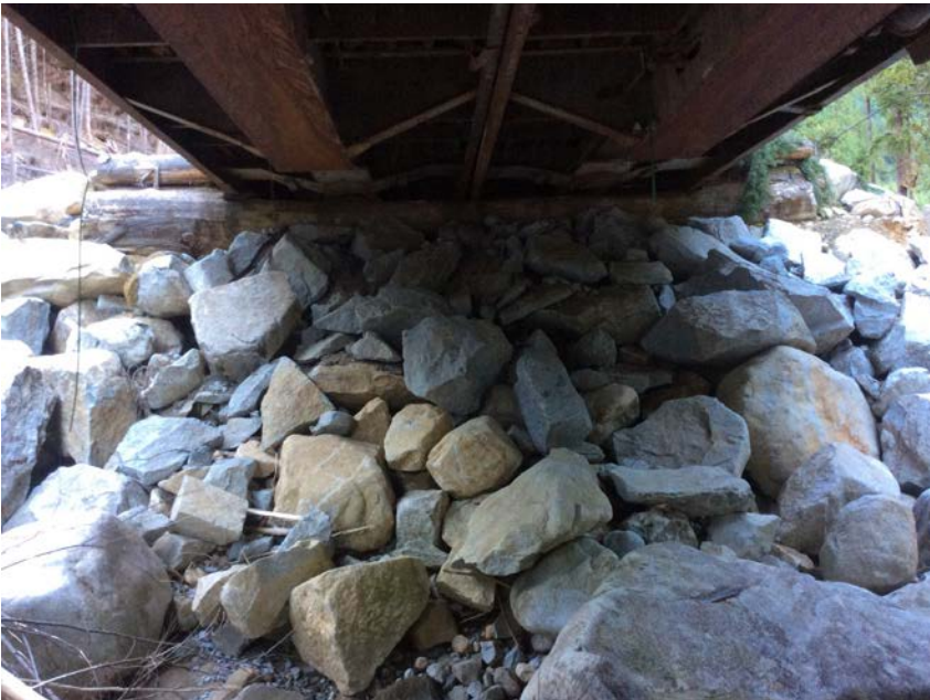
Left Bank Abutment when facing downstream
